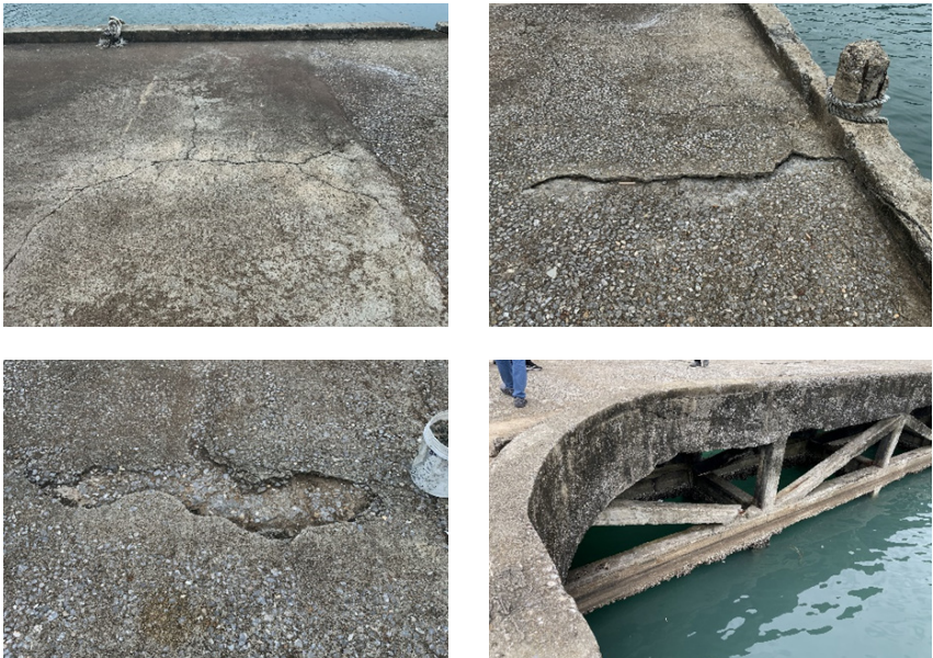
Visible surface cracks on the slabs and some columns.
